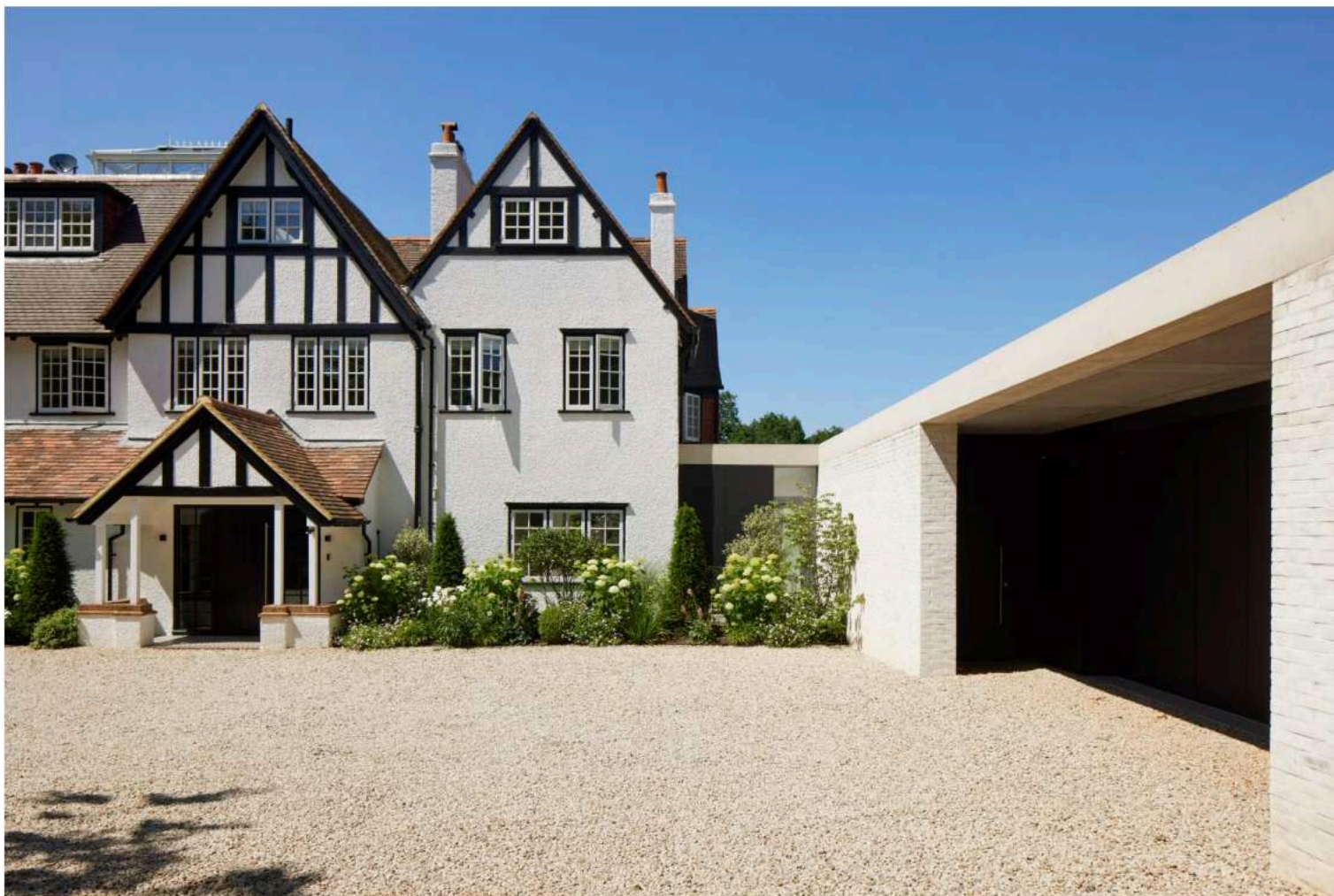
A garage was relocated to the front of the property
